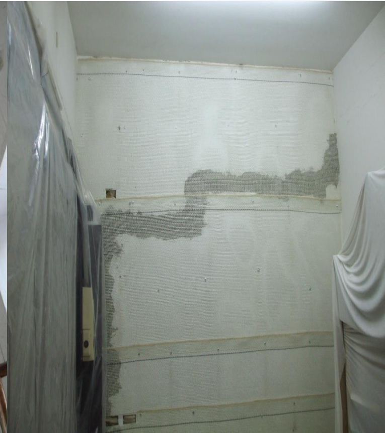
Repairing damaged house after earthquake
