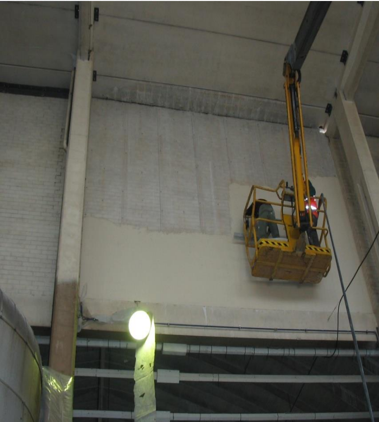
Fixing Industrial walls in a seismic area
