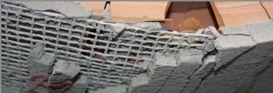
Figure 3 - Example of textile structure for earthquake containment 4
