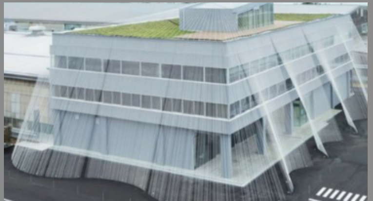
Figure 13 - The world's first earthquake resistant building strengthened by carbon fiber 8
